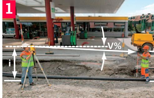
1 Setup and level the instrument on a point along the straight line the slope of which is to be determined. Position a staff at a second point along that line.
